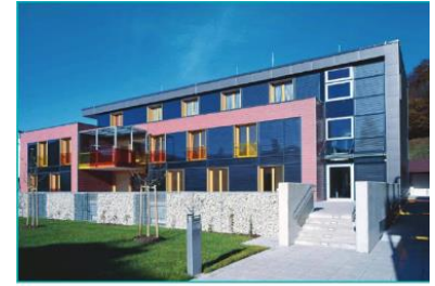
Figure 12 - Façade integrated flat-plate collectors in Austria. Source: DOMA
