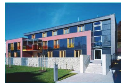
Figure 12 - Façade integrated flat-plate collectors in Austria. Source: DOMA
