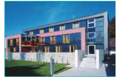
Figure 22 – facade integrated flat plate collectors in Austria Source: DGM
